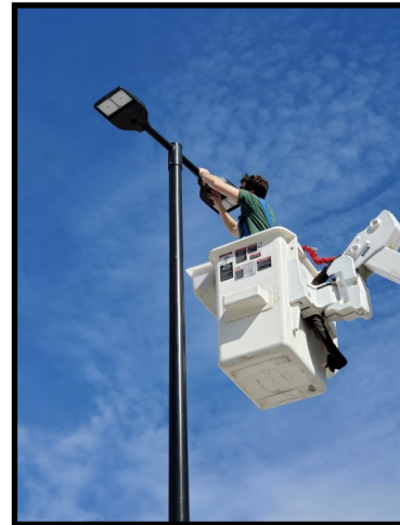
Campus Lighting Repairs
