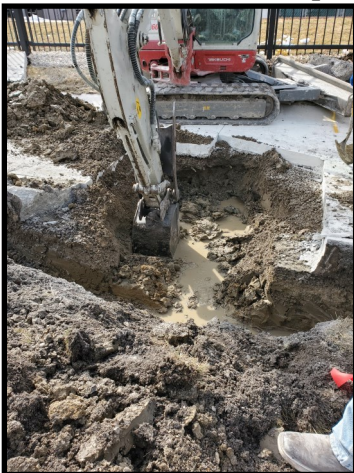
Stadium Water Line Repairs
